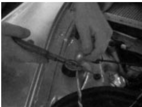
Running wires to the central control module.
